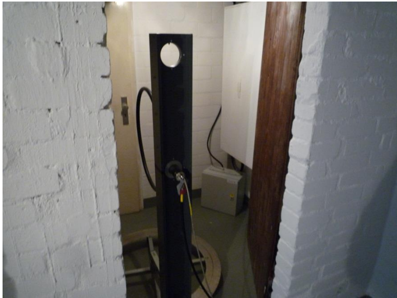
Figure 3 EMC measurements in the cellar beside the meter
