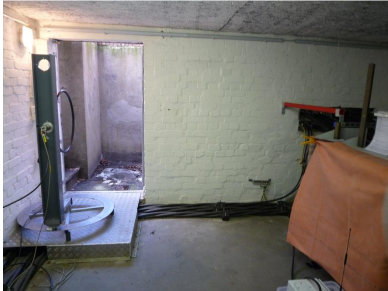
Figure 4 EMC measurements in a substation
